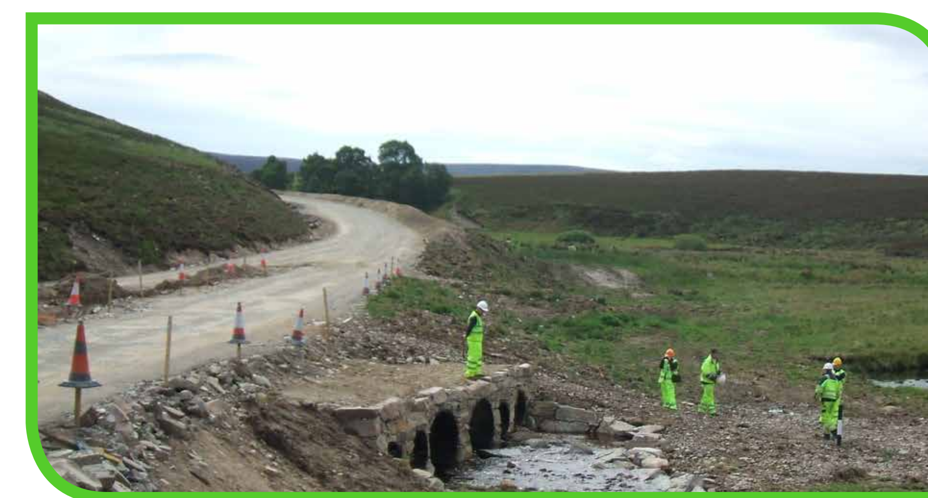
Careful design and maintenance of watercourse crossings (e.g. the depicted culvert in the onsite access track) is required to ensure that fish migration is not impeded.
