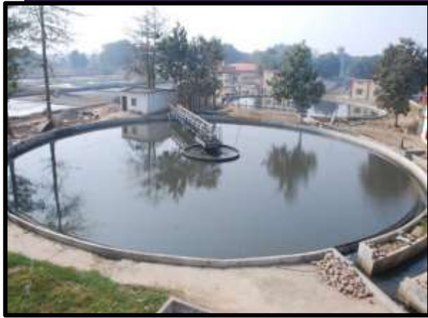
100% sewerage treatment infrastructure for 118 Towns
