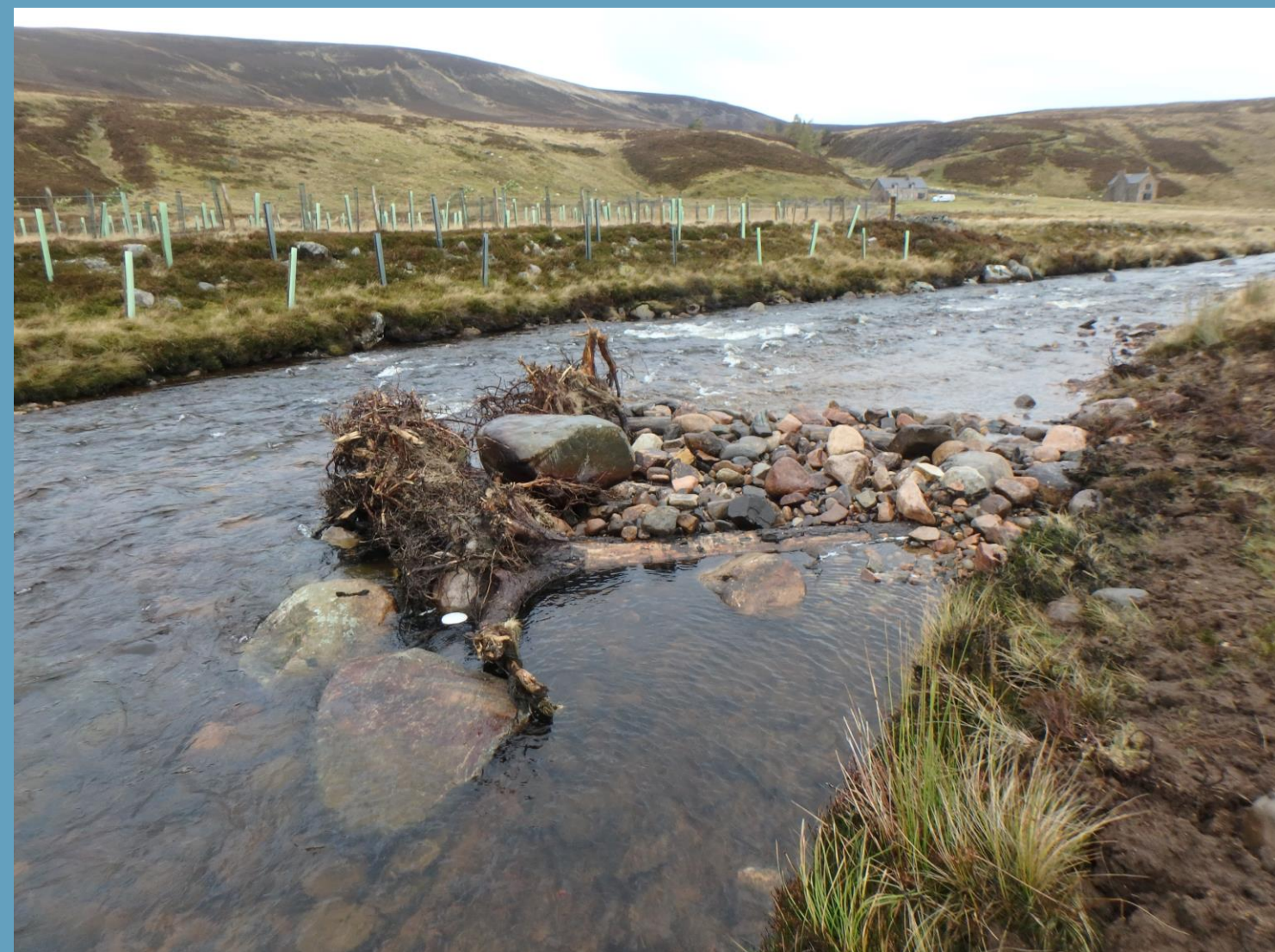
Figure 1 A lateral, bank attached LWS (LWS2) shortly after installation.
