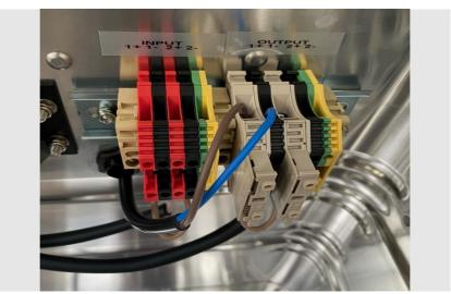
Figure 8: Terminal cabling for power supply
