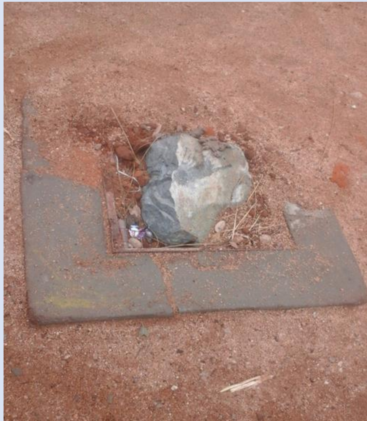
Figure 1. Image of a non-functional groundwater monitoring point in Machinga District. The monitoring point has been vandalised. (ND WASH Consultants, 2017)
