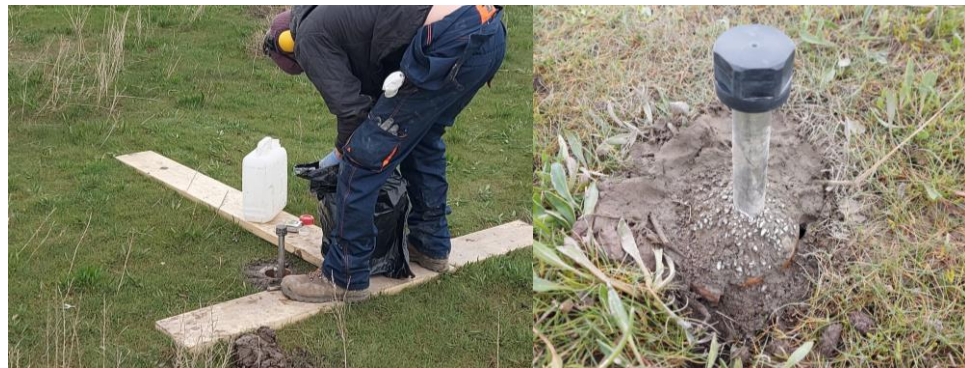
Setting the SET in with postcrete (Left). Installed SET base (Right).
