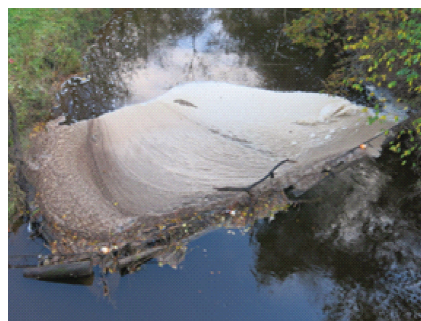
Scum and debris build-up
