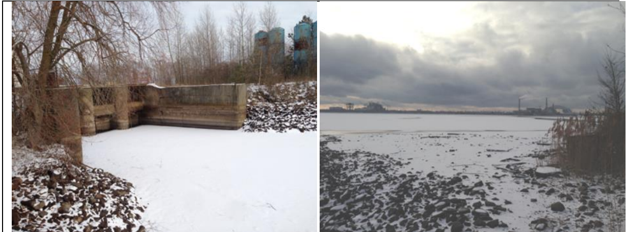
Fig. 2. Water level in the ChNPP cooling pond near the pumping station (BPS-3) in February 2015.
