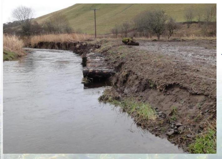
trees sufficiently deep  $\rightarrow$  less energy dissipation  $\rightarrow$  structure undercut and erosion of downstream bank
