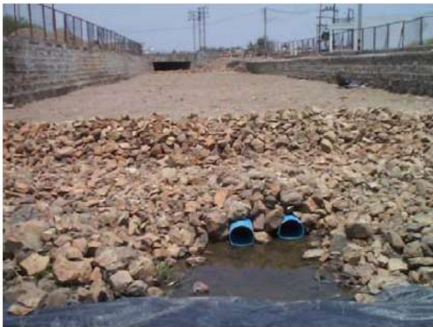
Pre-planted gravel bed for constructed wetland
