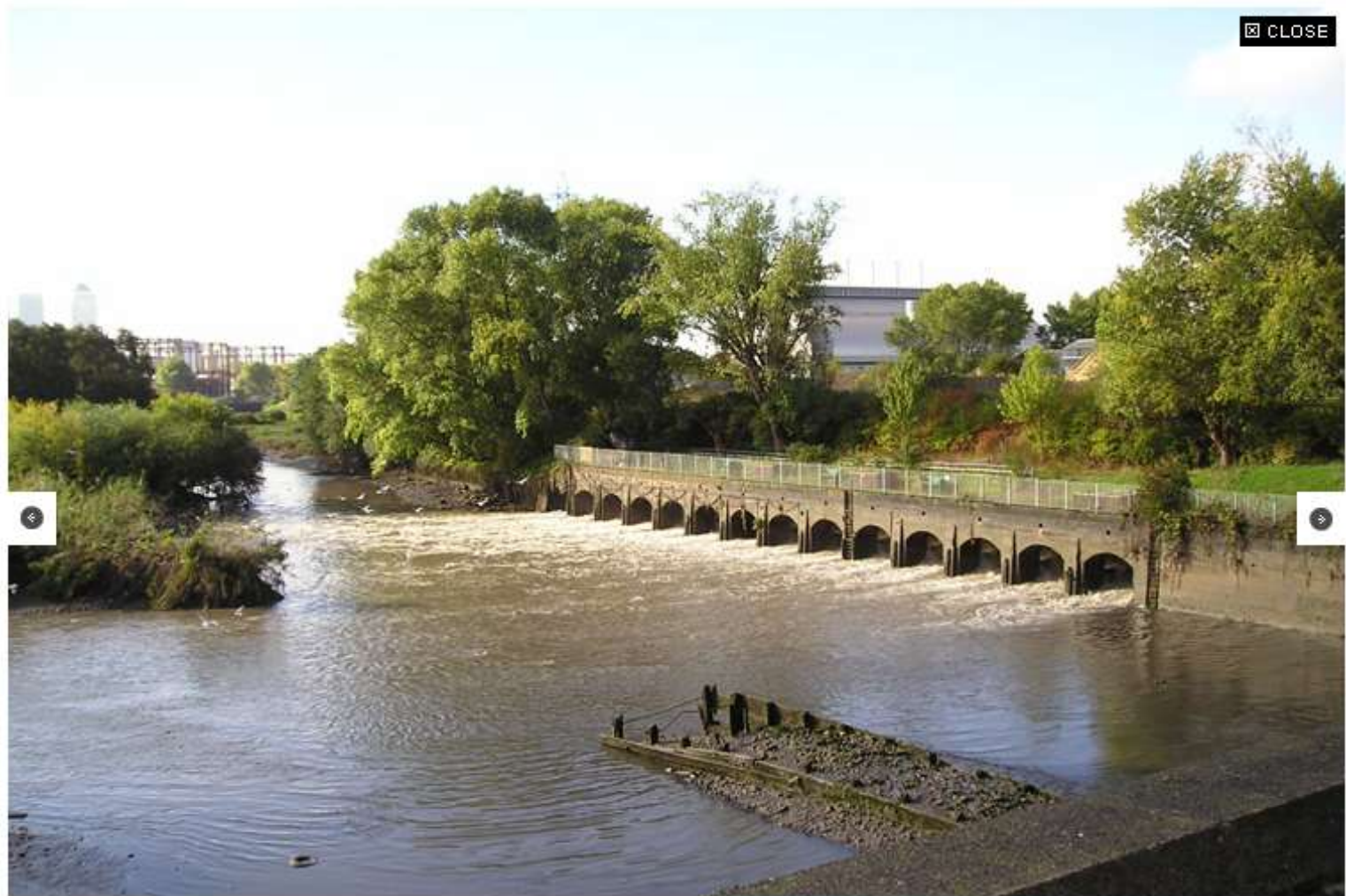
The largest combined sewer overflow (CSO) discharges into the River Lee from Abbey Mills Pumping Station. The Lee Tunnel will help prevent more than 16 million tonnes of sewage mixed with rainwater overflowing from this CSO each year.
